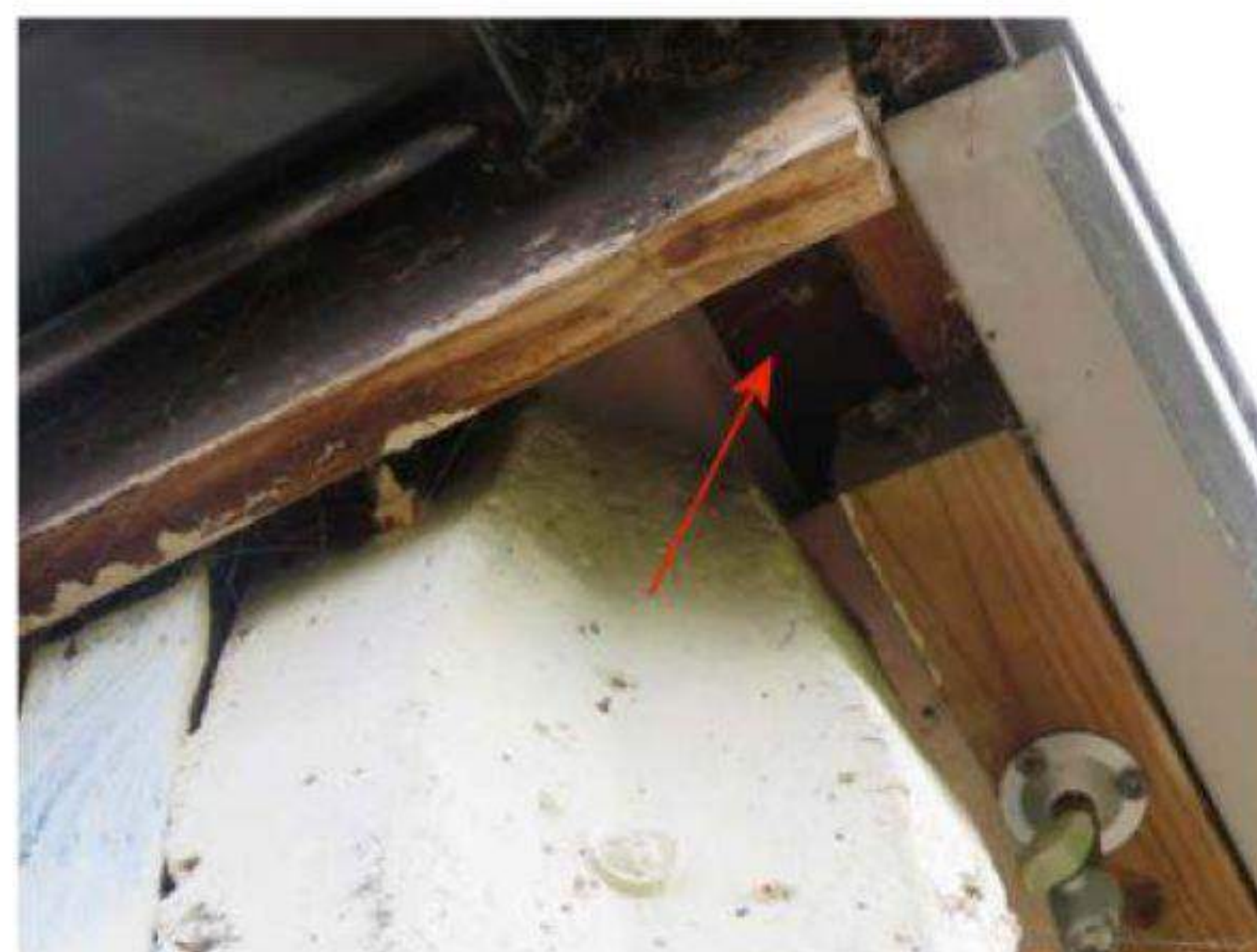
Photograph 29. Gap in the wooden soffit on the pavilion
