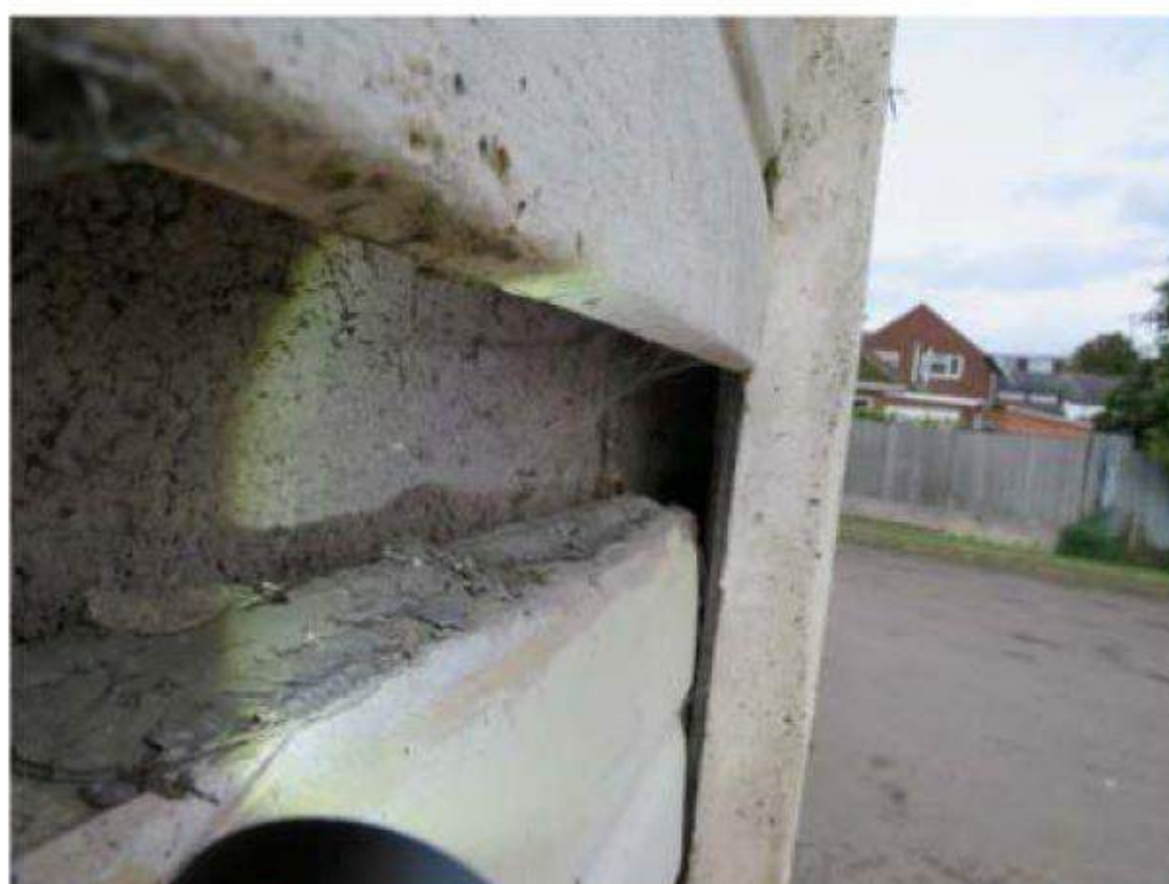
Photograph 28. Cavity between the block wall and the cladding on the pavilion
